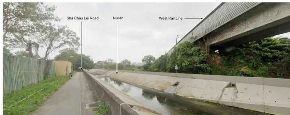
Existing Baseline Conditions
